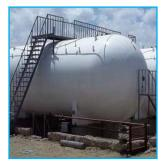
Spray irrigation of tanks aims to protect tanks and other vessels against unacceptable heating during burning. Here, heating must be understood as a condition where an increase of a tank's inner pressure and a decrease of the tank walls' resistance will lead to bursting of the tank.
